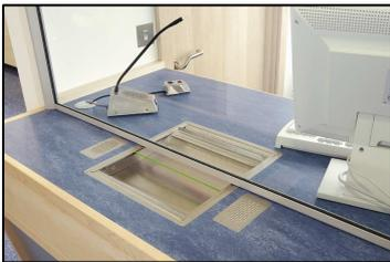
**3: Flush Mounting System with Loop Facility**
