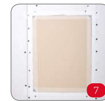
7 For drywall applications only, set panel back 1mm to 2mm from front wall. Fill joint and skim surface with Easi-fill lightweight repair plaster.
