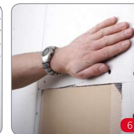
6 Apply joint tape, covering joint between panel and plasterboard. Perform final electrical/audio test.
