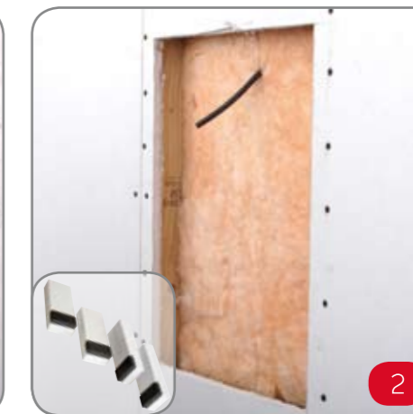
2 Position installation lugs under top and bottom corners of surrounding plasterboard. Ensure cables are pulled to this position.
