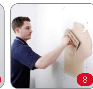
8 Skim with plaster (ordinary multifinish is fine). The best finish is produced when the entire wall is skimmed at the same time. Allow plaster to dry thoroughly before using and before decorating with paint or wallpaper.
